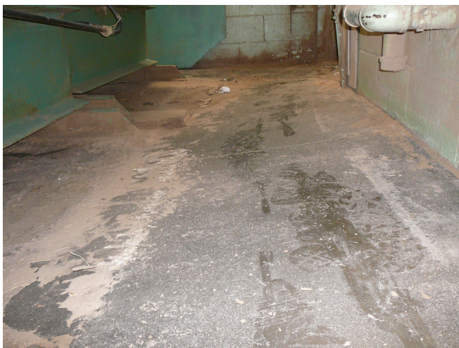
Photo 13. Significant settlement of slab on grade in an industrial building.
