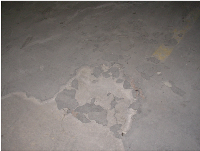
Photo 9. Polyurethane membrane on suspended slab of parking garage is wearing off.
