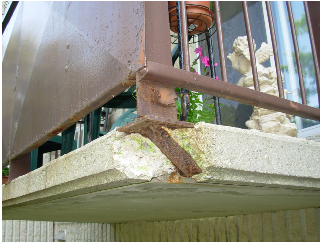
Photo 11. Typical corrosion of steel anchor embedded in concrete balcony slab, causing concrete to spall.
