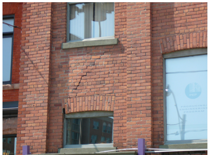
Photo 14. Typical settlement cracking in solid masonry wall of an older downtown building.
