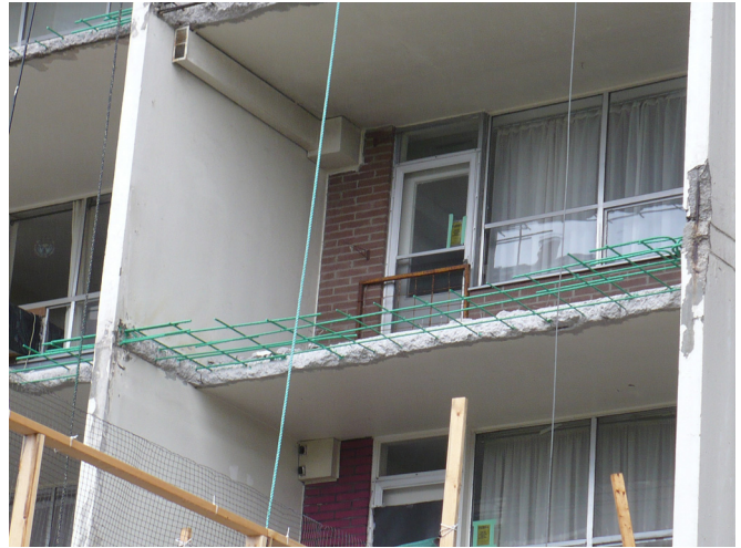
Photo 10. Slab edge repairs being undertaken to balconies. Note the new steel rebar is epoxy coated.
