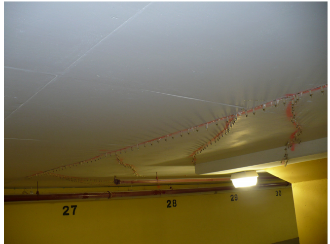
Photo 12. Numerous epoxy injection repairs to cracking in underside of suspended slab of parking garage.
