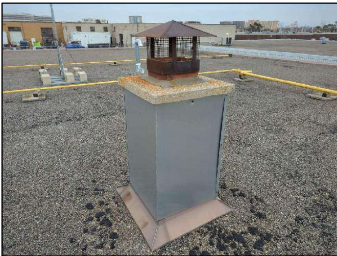
Photo 26. Masonry chimney covered with metal cladding at the upper level roof.
