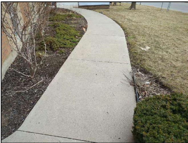
Photo 17. Concrete sidewalk at main building entrance.
