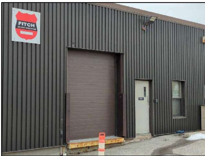
Photo 8. Loading dock overhead door.
