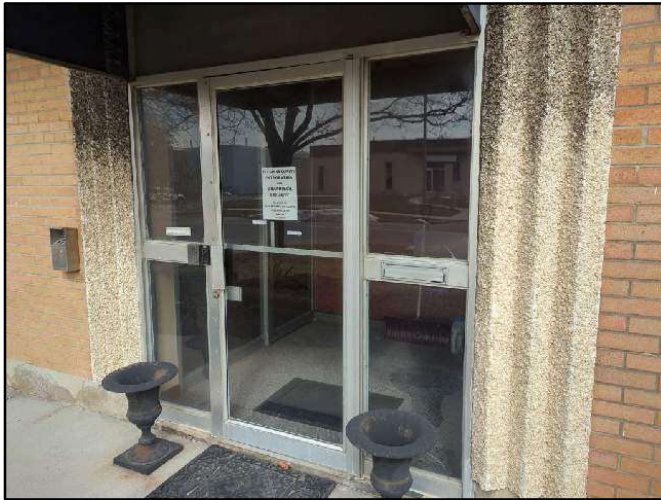
Photo 7. Main entrance door.
