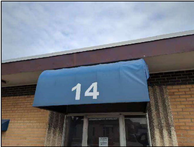
Photo 28. Steel-framed front entrance canopy.
