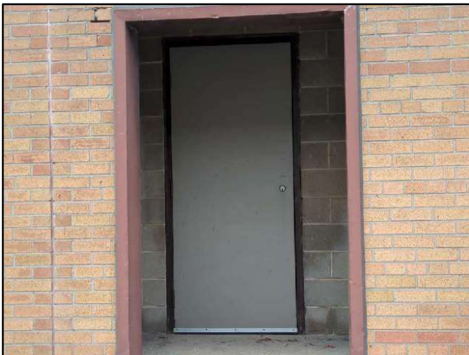
Photo 6. Typical exit door.
