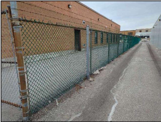
Photo 16. Typical perimeter fence.
