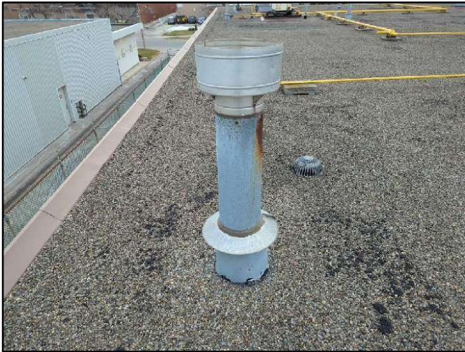
Photo 25. Metal chimney at the upper roof level.
