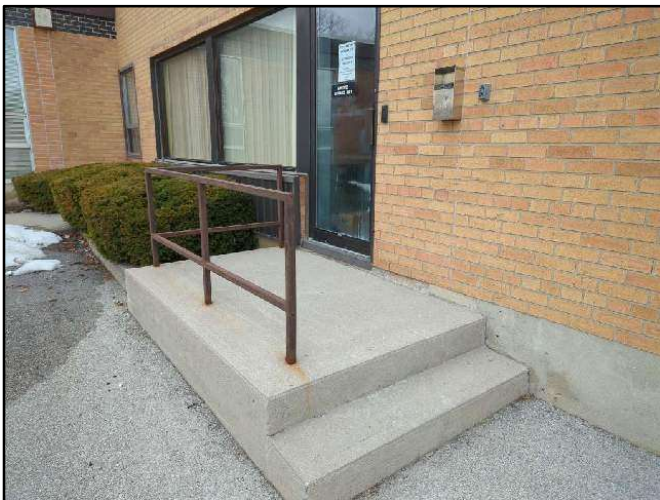
Photo 20. Poured concrete steps at the southeast exit.
